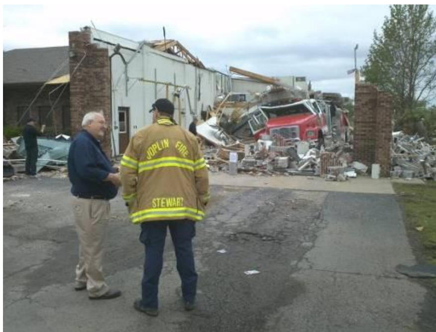
Figure 5: FEMA Administrator Craig Fugate surveys a damaged fire station with a Joplin firefighter. (Source: FEMA)
