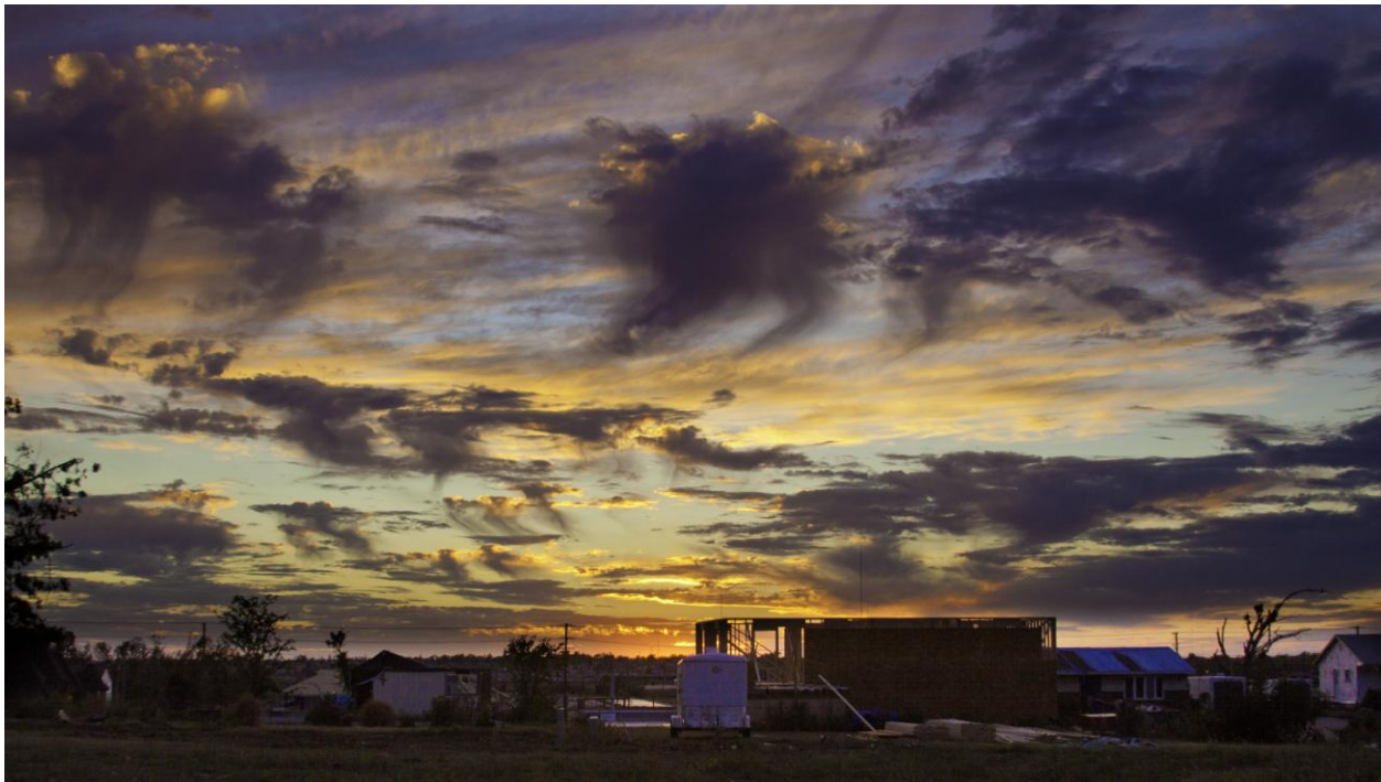
Figure 1: New home construction in Joplin, September 2011. (Source: FEMA)
